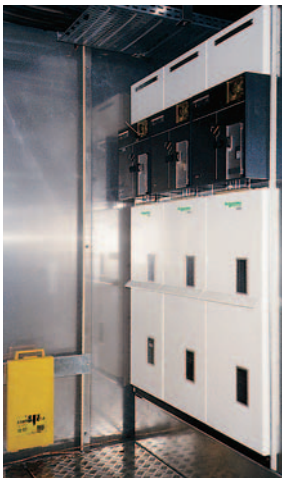
Installation of 400 - 630 A units on a 350 mm plinth
